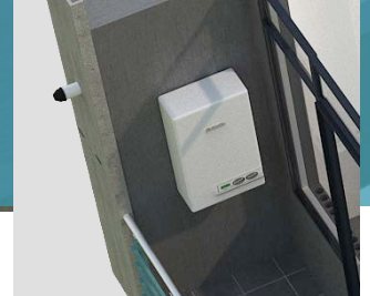
Boilers linked to the central heating system
